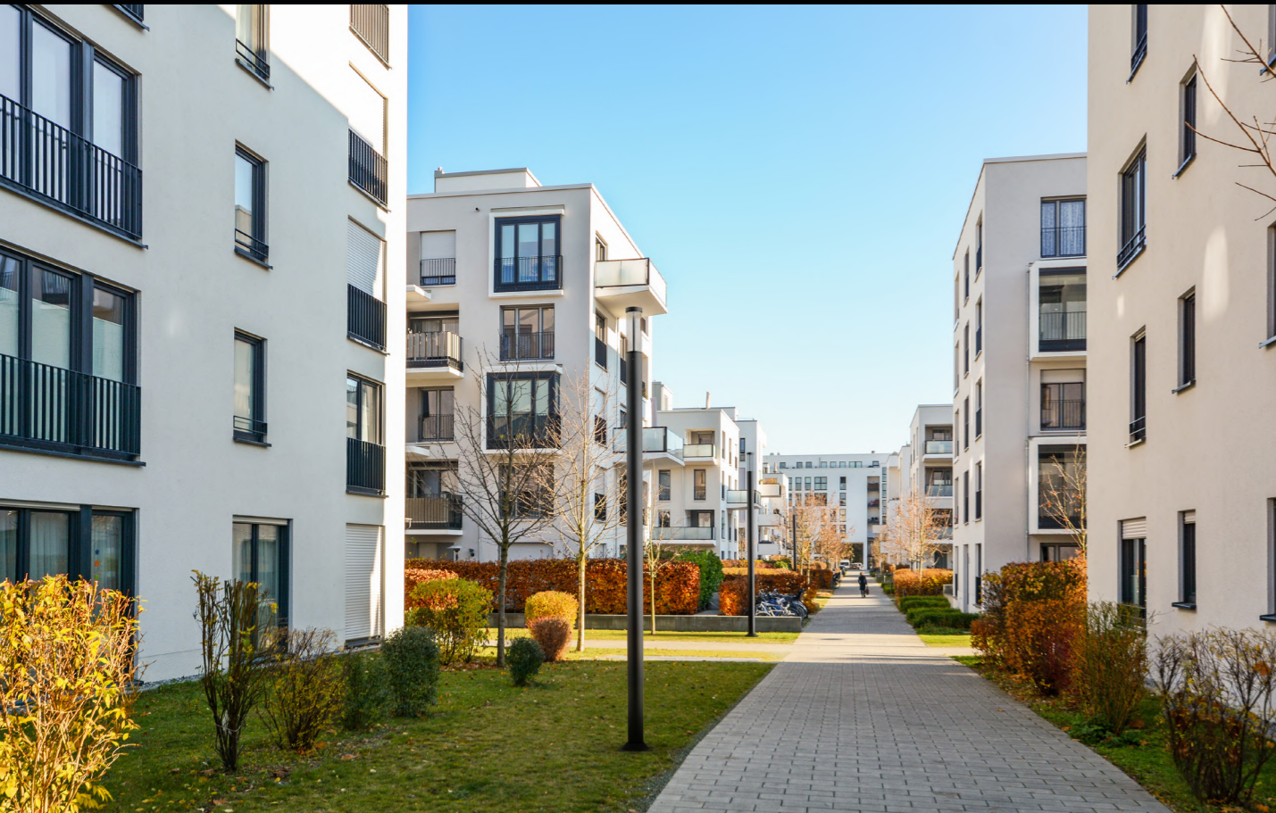
With its plain look and low glare optics, VLORA is a reliable choice for exterior site lighting applications.
